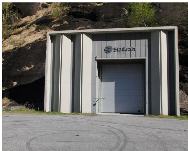
Entry Grytten hydropower plant (photo Statkraft)
