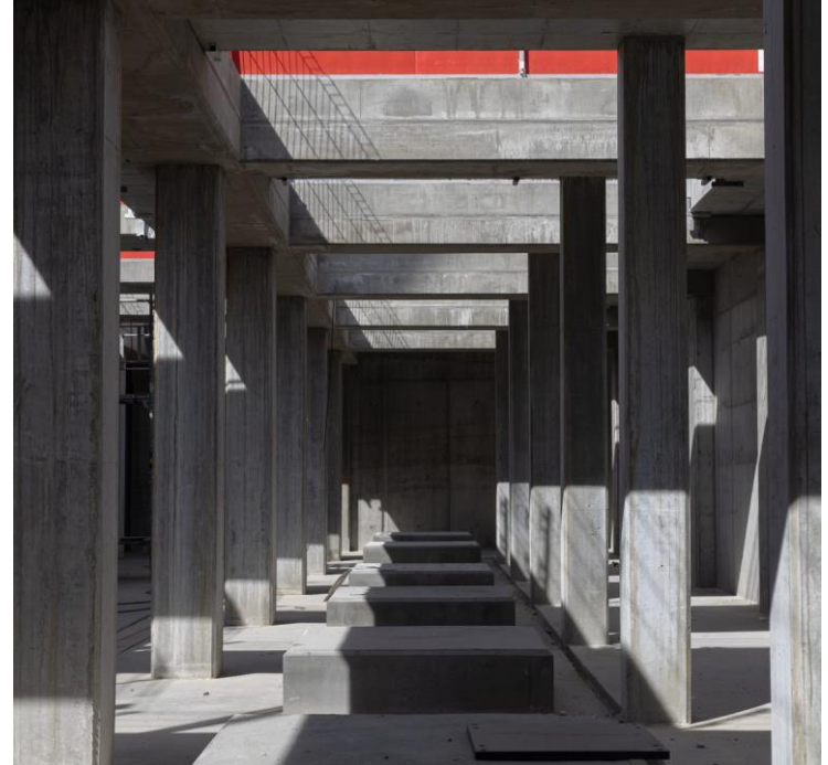
Concrete work on water intake station almost completed
