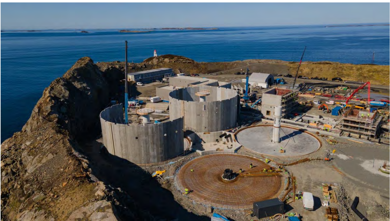
Indre Harøy drone picture April 2021
