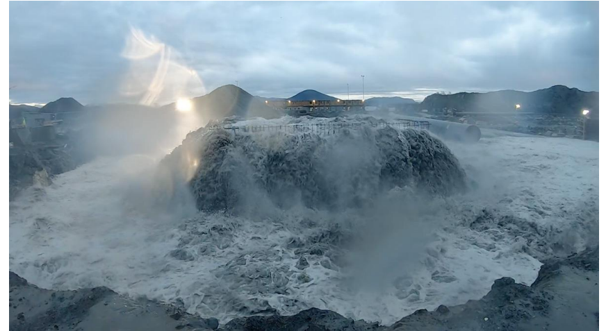
Blasting work for wastewater tunnel
